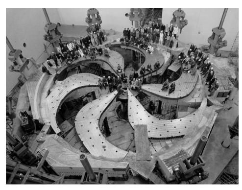
TRIUMF cyclotron magnet (1972): 500 MeV protons.
