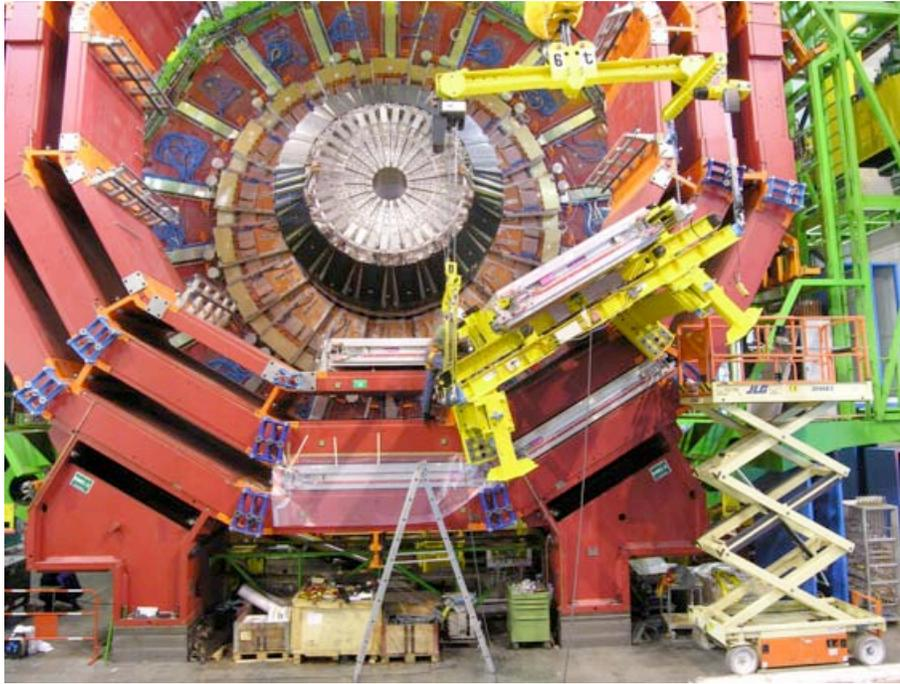
Figure 158: Installation of MB1 station on Wheel -2. The yellow frame is the *cradle* used to insert the chamber in its location inside the iron slot.
