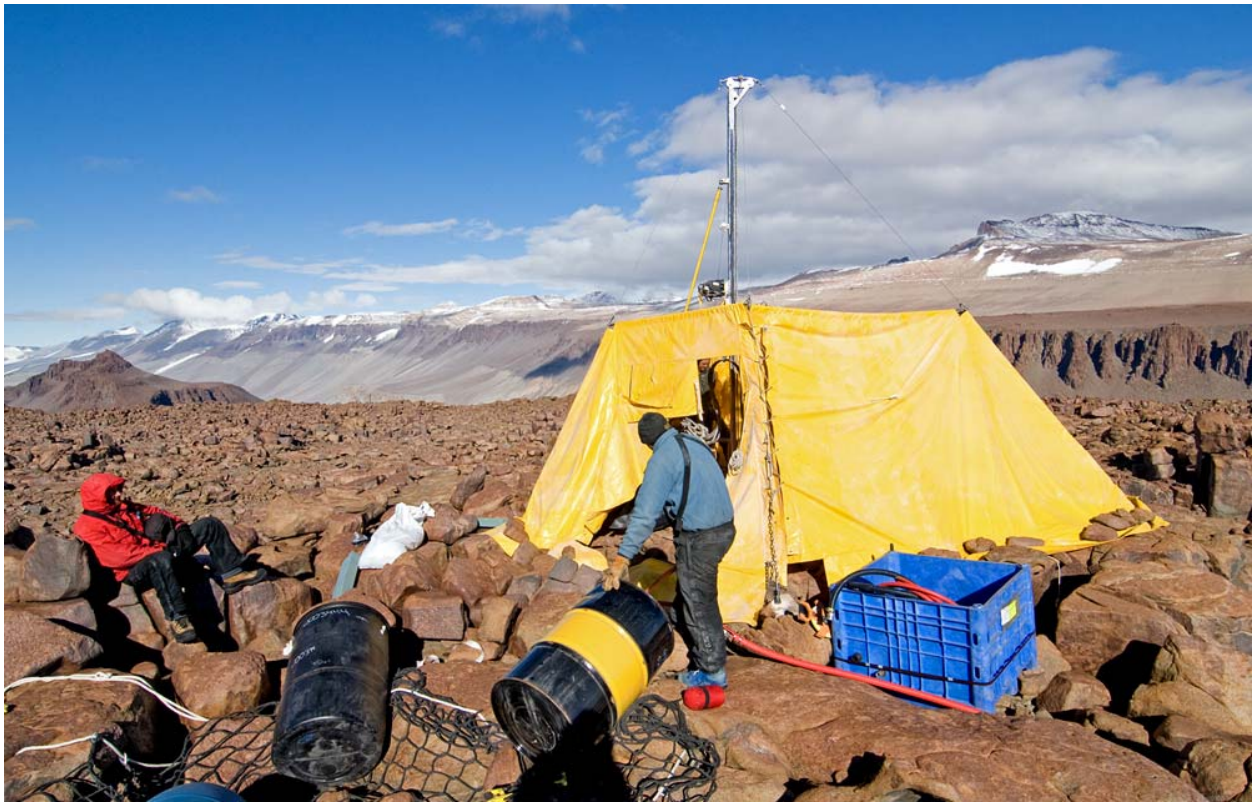
Setting up the drill and fluid circulation system at The Labyrinth (dolerite) site.
